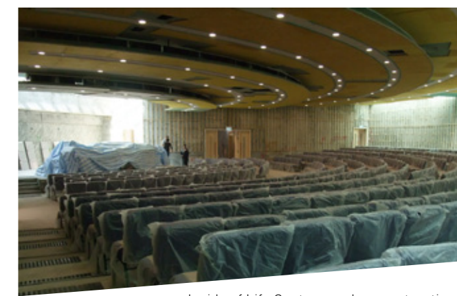
Inside of Life Centre - under-construction
