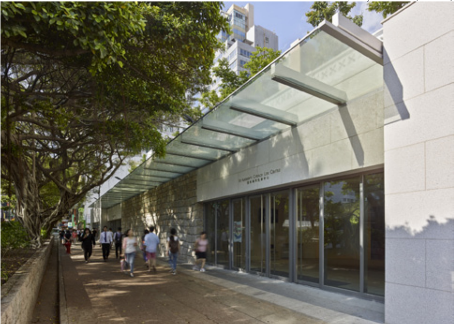
South Lobby Entrance (Bottom)
