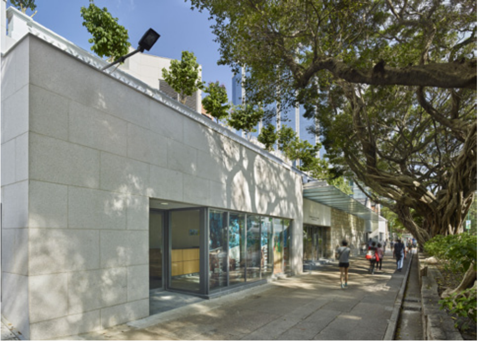
North Lobby Entrance (Above)
